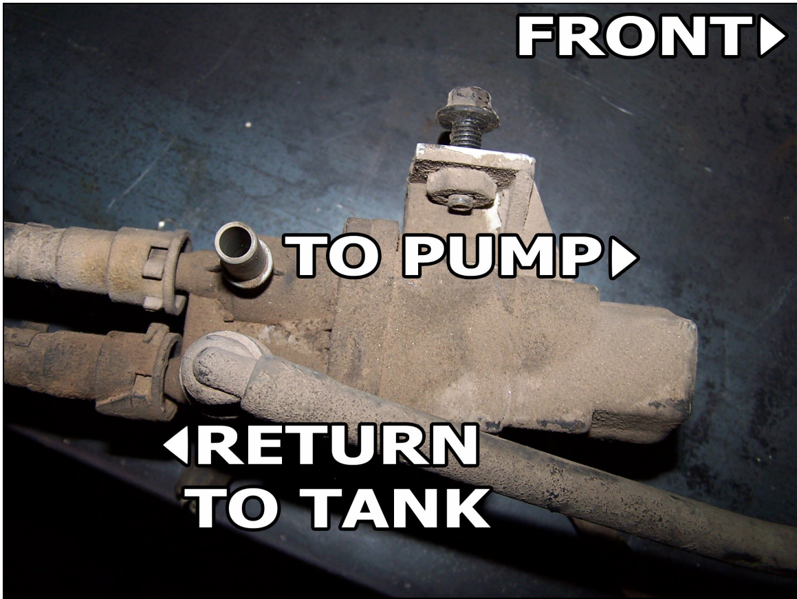
Figure 5 – Fuel Tank Selector Valve – RETURN HOSE Identification
